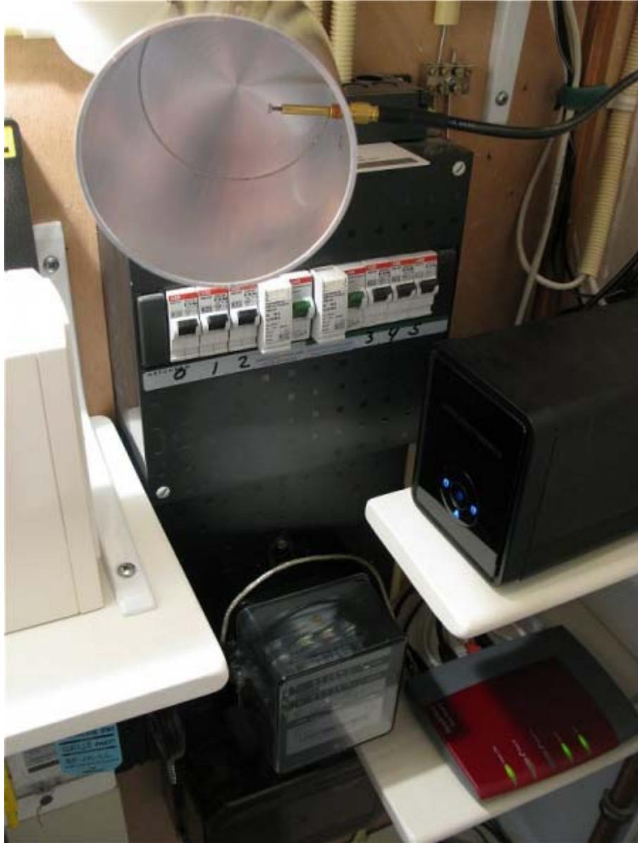
Here is the new situation! Bottom right you see the Fritz!Box with its new antenna cable. The antenna now has a much better and higher position, radiates in the right direction, and the radiated energy is not absorbed by its surrounding metals!
